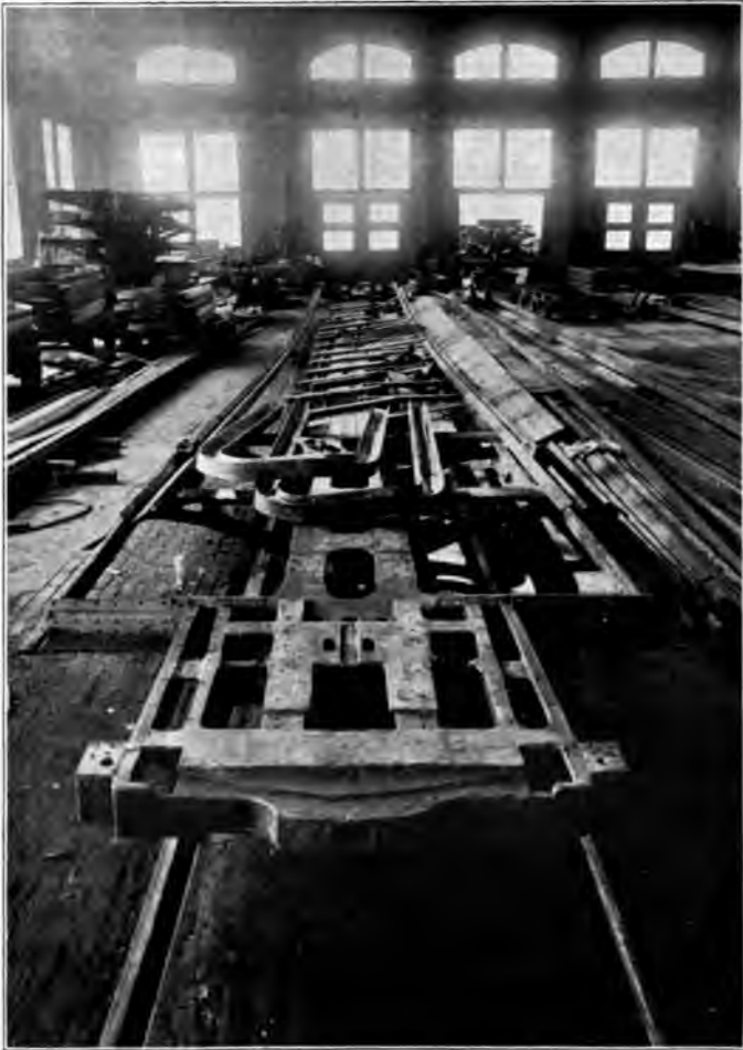
The first step in the building of the car. The center construction in position, and the framework assembled
